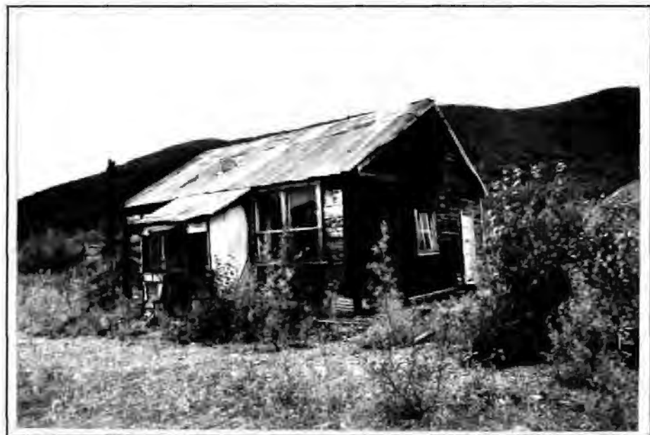
Figure 153. The Bunkhouse at the Discovery/Peter Miscovich Camp, 1993. The view is looking northwest.
